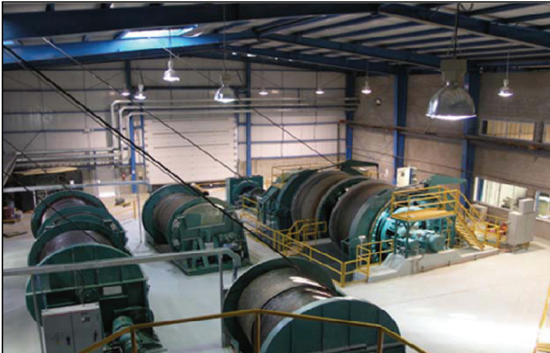
Figure 9-3: Typical Shaft Hoist House
